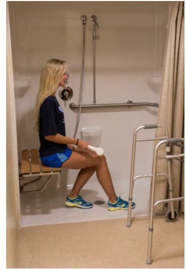
Shower modifications: handrail, stool, adjustable shower
